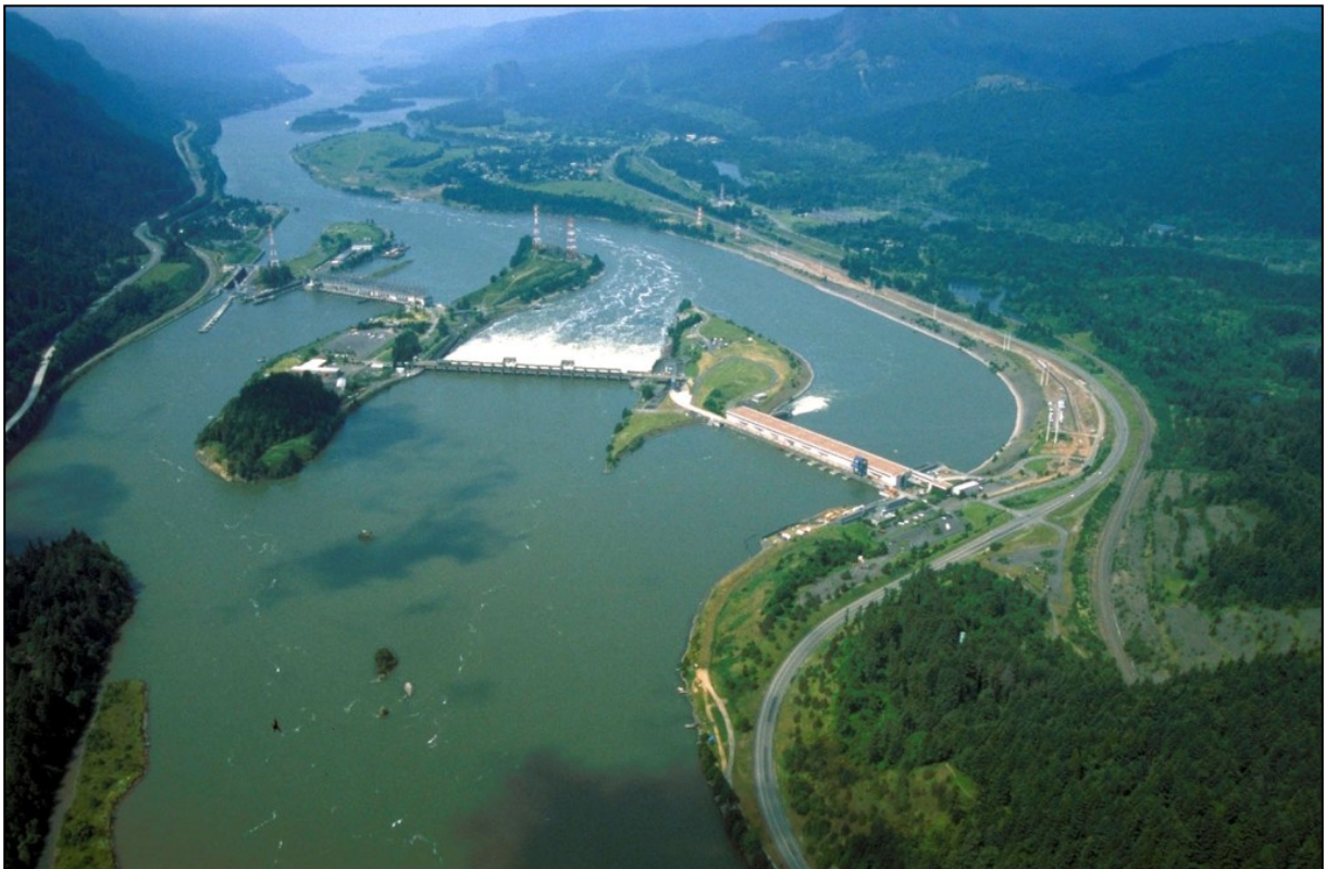
Bonneville Lock and Dam
